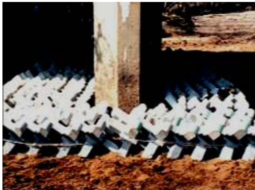
Figure 21: A-Jacks protecting bridge pier
