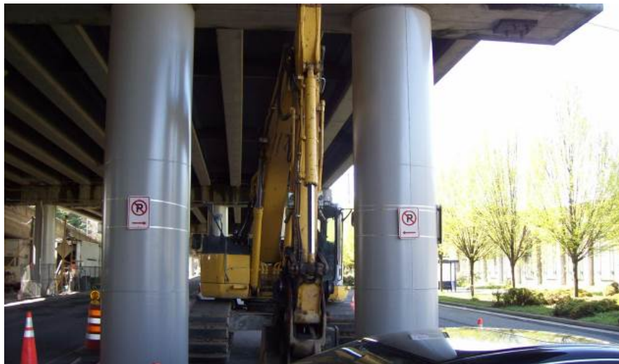
Figure 25: Jacketed bridge pier
