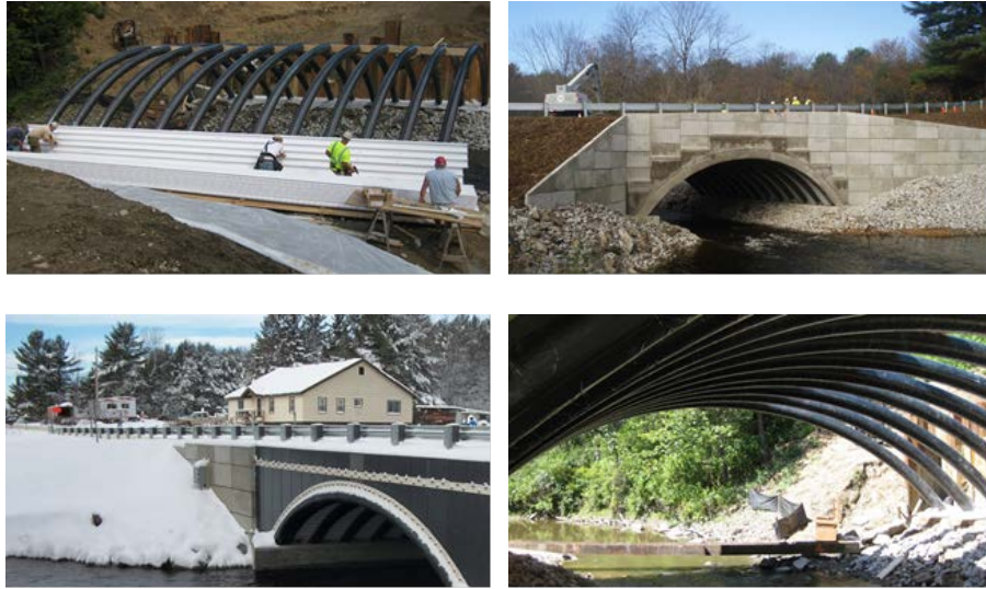
Figure 51: Bridge in a backpack
