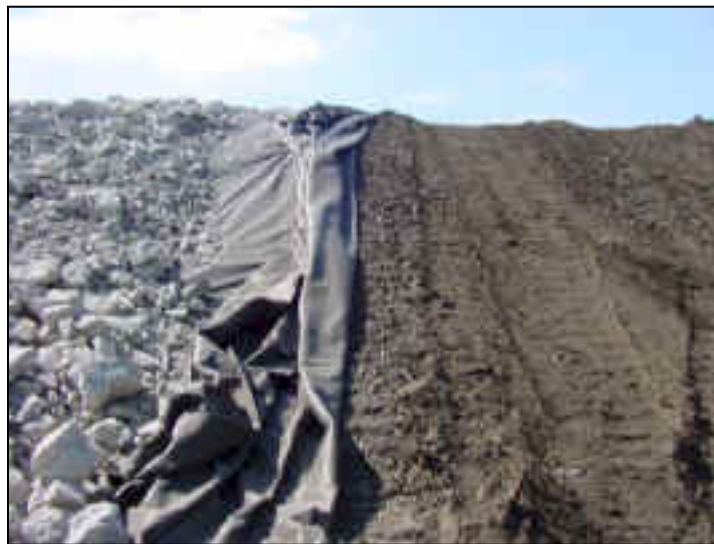
Figure 46: Soil covered by filter fabric is then covered with rip-rap
