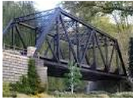
Figure 14: Steel truss bridge
