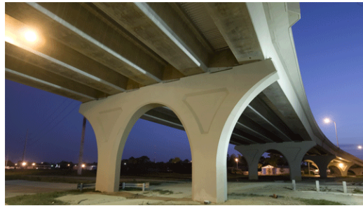
Figure 37: Bridge built with HPC
