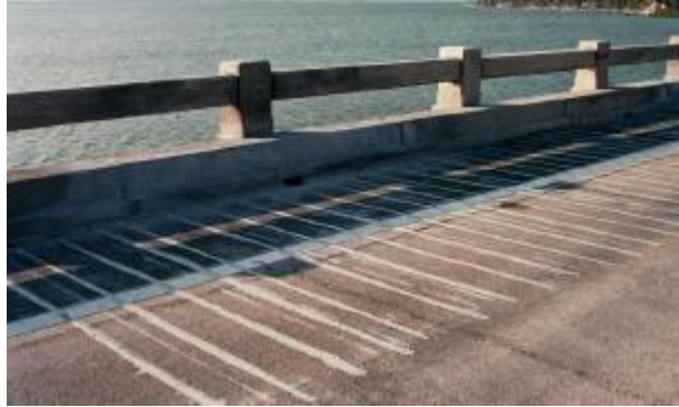
Figure 8: Reinforced bridge deck slab
