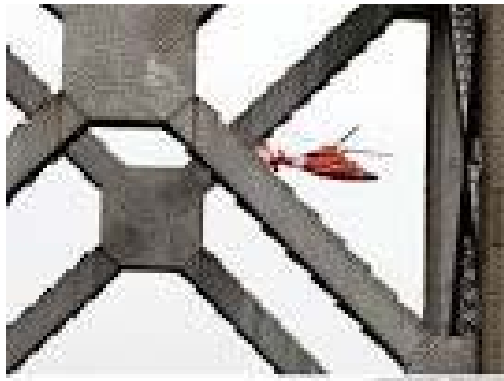
Figure 53: Bridge boxed lattice
