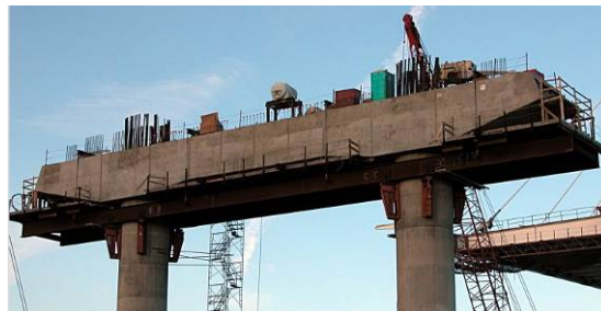
Figure 26: Capped bridge pier
