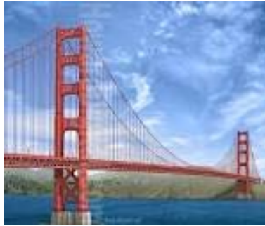
Figure 11: Golden Gate cable suspension bridge
