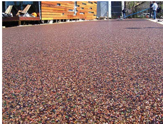
Figure 19: Asphalt mixed with glass
