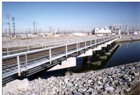
Figure 15: Open deck bridge
